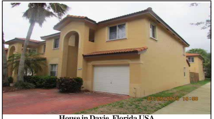
House in Davie, Florida USA
