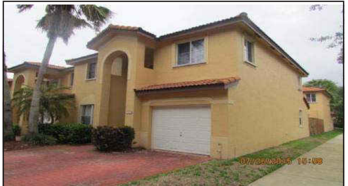
House in Davie, Florida USA
