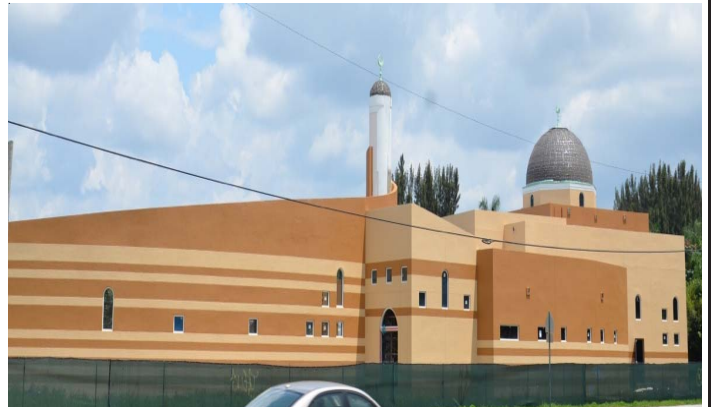
Photo Above: Al-Amin Center Construction Development
