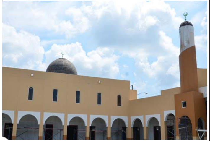
Photo Above: Al-Amin Center Construction Development
