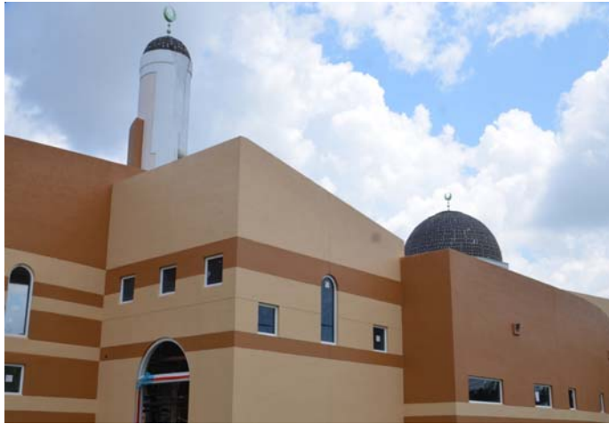
Photo Above: Al-Amin Center Construction Development
