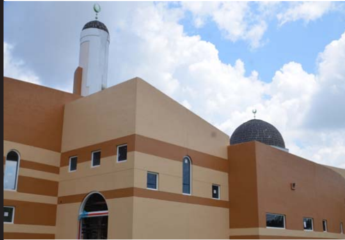
Photo Above: Al-Amin Center Construction Development
