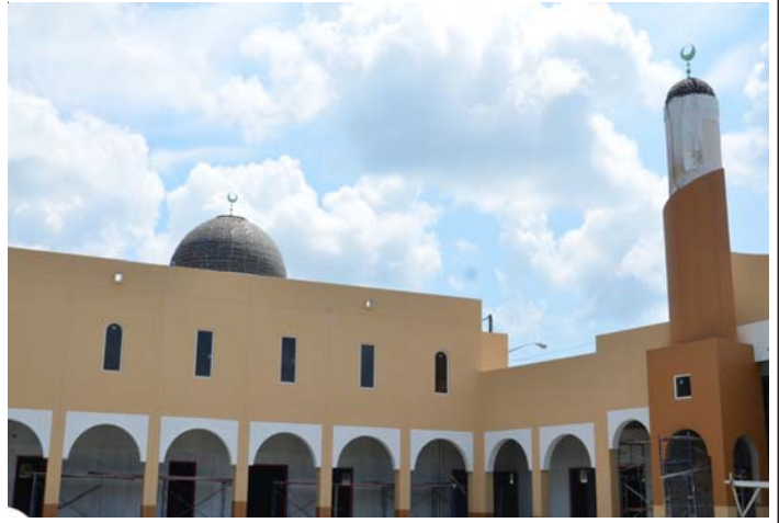
Photo Above: Al-Amin Center Construction Development
