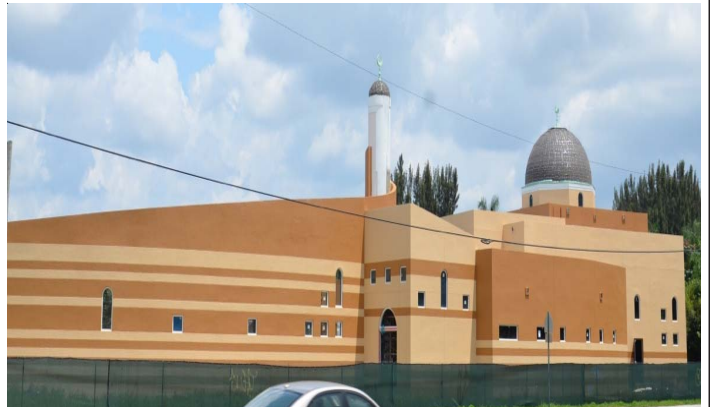
Photo Above: Al-Amin Center Construction Development
