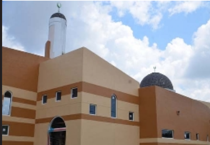
Photo Above: Al-Amin Center Construction Development
