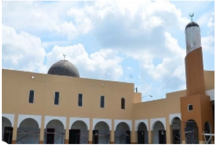
Photo Above: Al-Amin Center Construction Development
