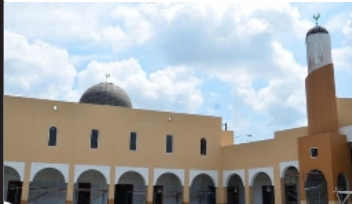
Photo Above: Al-Amin Center Construction Development
